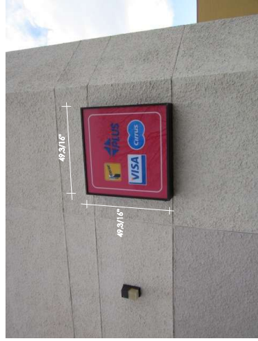
Approximated View of Existing Sign
